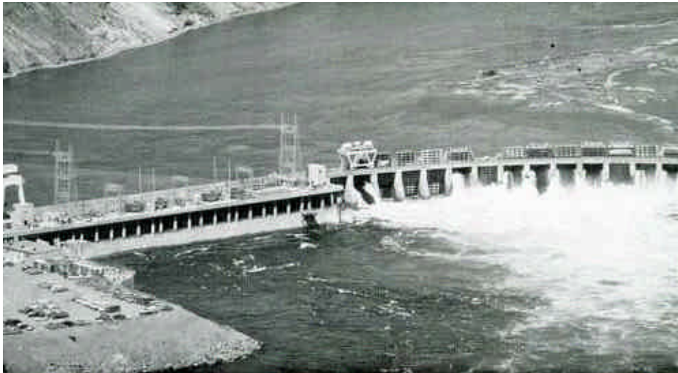
Figure 1: Aerial view of spillway and Powerhouse Two at Rock Island Dam.
