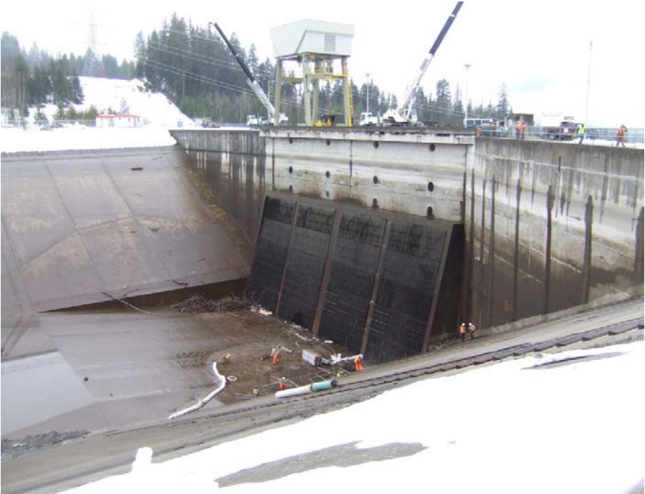
Figure 4 Picture of the intake after de-watering showing trapezoidal channel.
