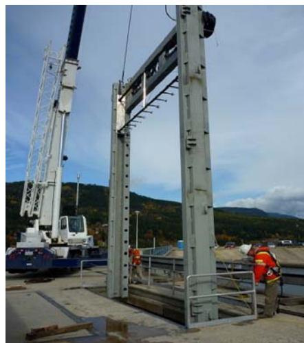
Figure 6: Transducer support frame being deployed into the gate slot.
