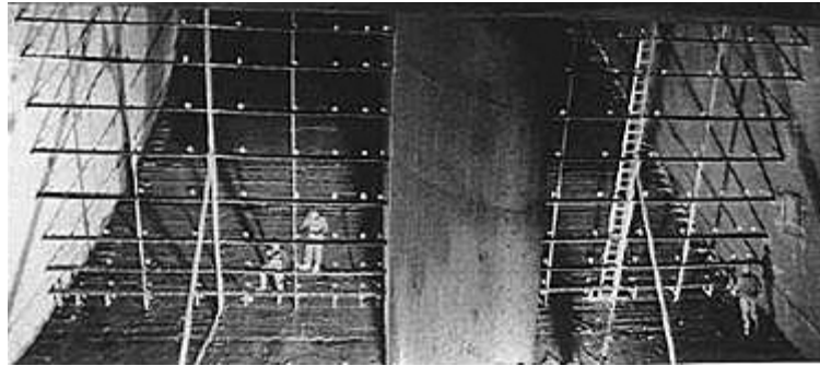
Fig. 2 – Current-meters at Formin plant (courtesy Turboinstitut - IGHEM 1996)
