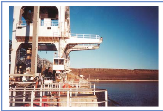
McNary Dam (U.S. Army Corps of Engineers)
