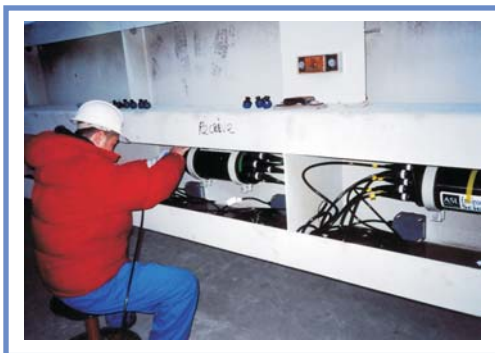
Installing equipment on ASFM frame
