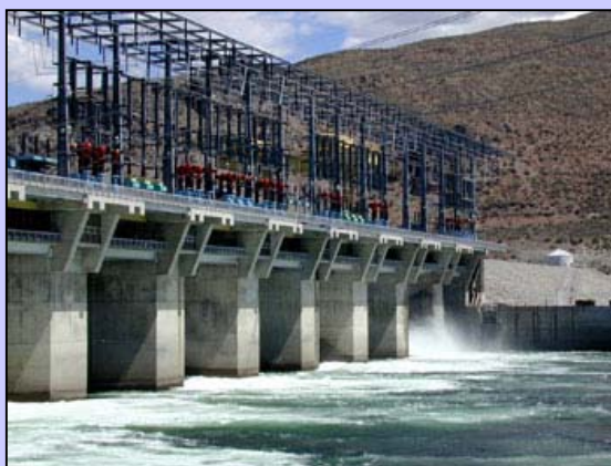
Photo courtesy Douglas County PUD
